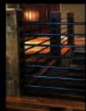
balustrade to raised area
