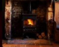
new stove to existing stone chimney
