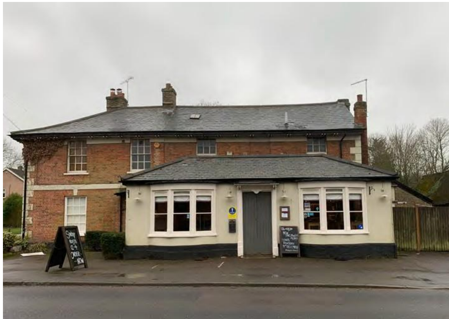
EXISTING EXTERNALS TO PUB
